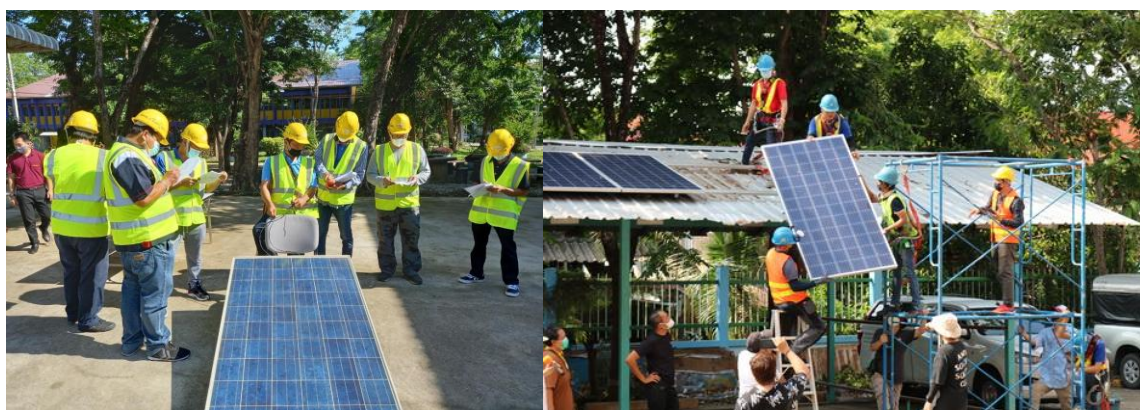
The Nonthaburi Provincial Skill Development Department provides training on the installation of photovoltaic (PV) solar panels.
